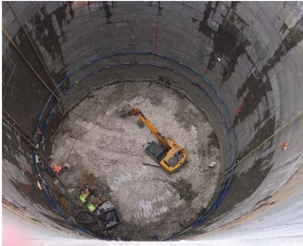
In-shaft wellpoint system, chalk exposed
