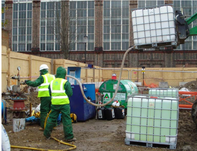
Acidisation of a chalk well with HCl
